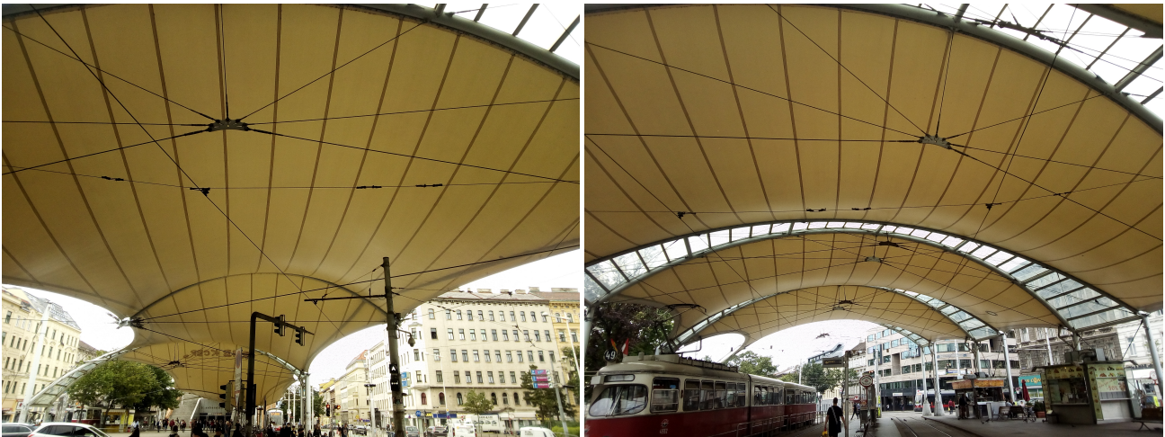
Figure 1.1: An example of a tensile membrane structure, a tram station roof in Vienna, Austria.
